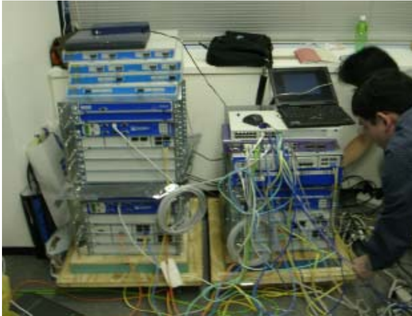
Core routers (Juniper M20), And Router testers
